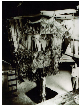
Fig. 1 The Spanish architect Gaudi used an articulated model of a cathedral suspended upside down to help in its design. This could also be seen as an attempt to capture the spiritual sense of 'grace', that is, whatever stands in opposition to 'gravity' (I have borrowed these terms from the philosopher Simone Weil). (Photo courtesy of Aplicaciones y Reproducciones Mas).
